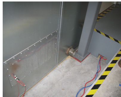
FIGURE 4. A penetration panel sits below the building floor, providing access to cables that run under the chamber's raised floor. A pipe opening alongside the panel provides access for additional cables and hoses.
